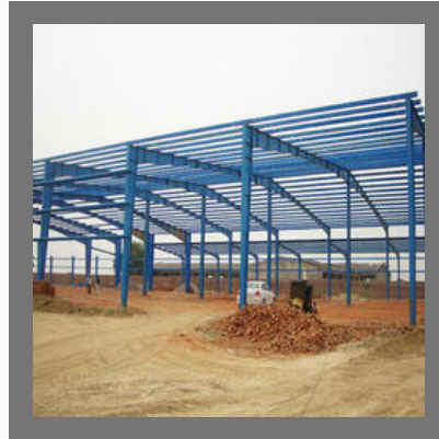
Pre Engineered Structure
