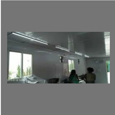
Rooftop Porta Cabins
