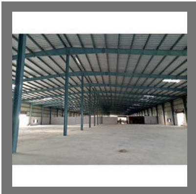
Galvanized Mild Steel Industrial Shed
