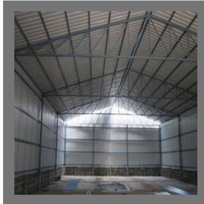
Mild Steel Industrial Shed
