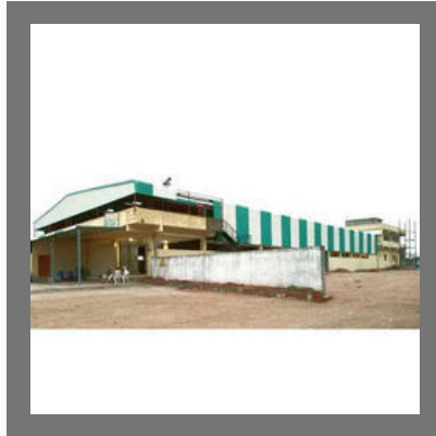
Pre Engineered Steel Building
