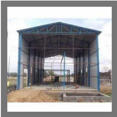
MS Shed Fabrication
