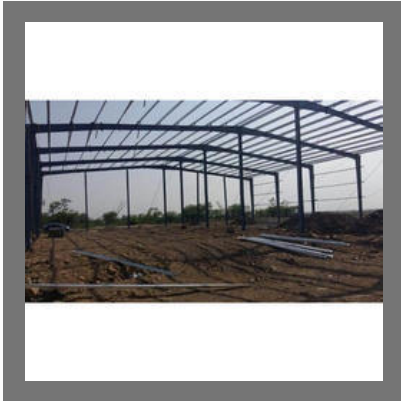
Pre Engineered Building Structure
