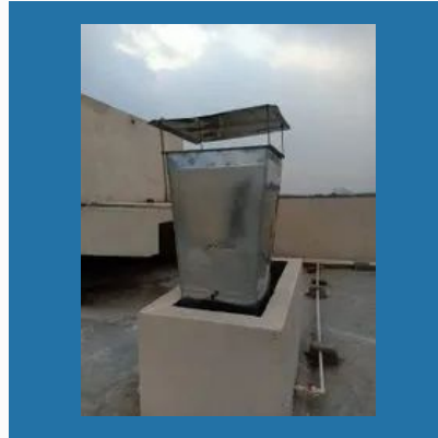
Ss Industrial Chimney
