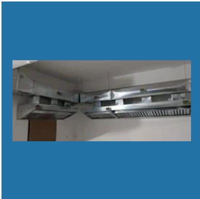
Hotel Ducting work
