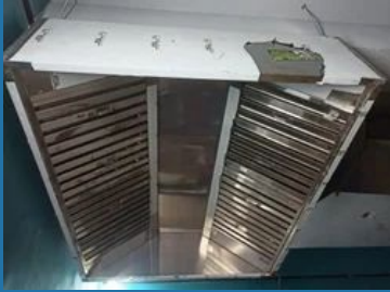
Kitchen Exhaust Hood
