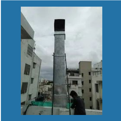
Duct Cleaning Services
