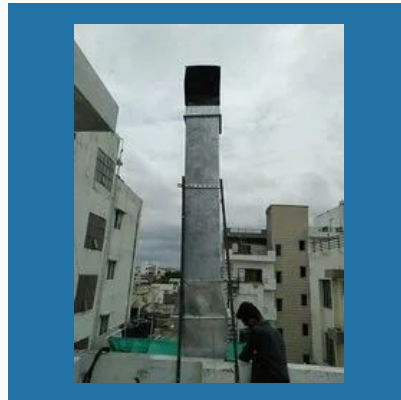
Industrial Ducting Works
